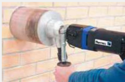
Messa in opera
